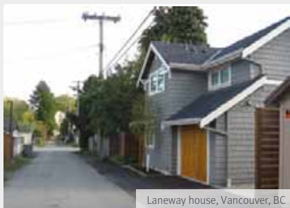
Laneway house, Vancouver, BC
