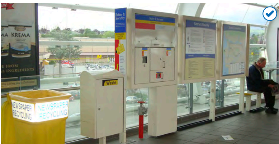
Use of standardized platform furniture module. Millennium Line, Burnaby.
