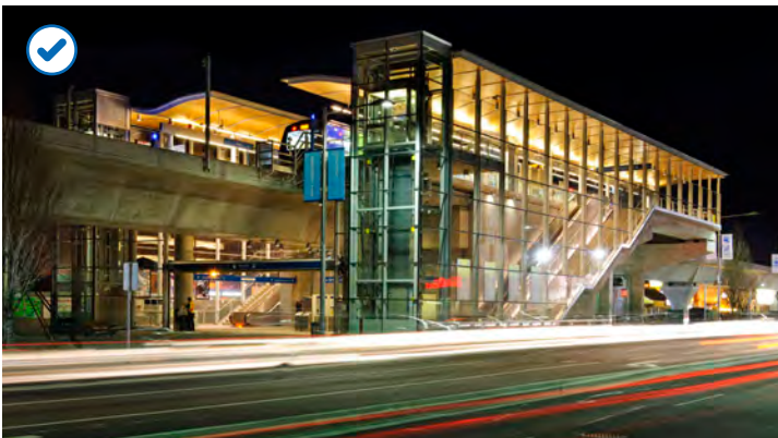
Transparency and high quality lighting connects interior and exterior spaces. Aberdeen Station, Richmond.
