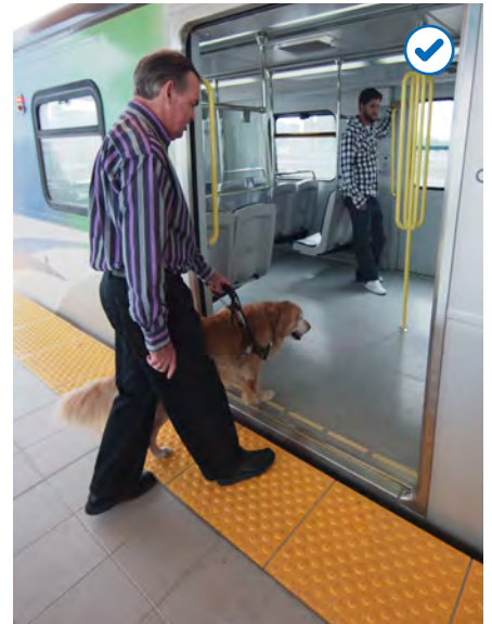
Platform edge high-contrast, tactile warning strip. Canada Line, Vancouver.
