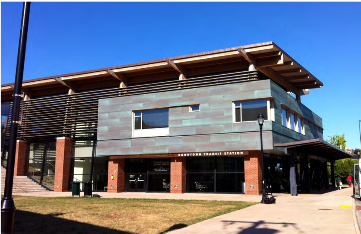
South and west elevations showing the deep wooden canopy shielding the building from solar heat gain and louvred windows wrapping the second floor to manage glare.
