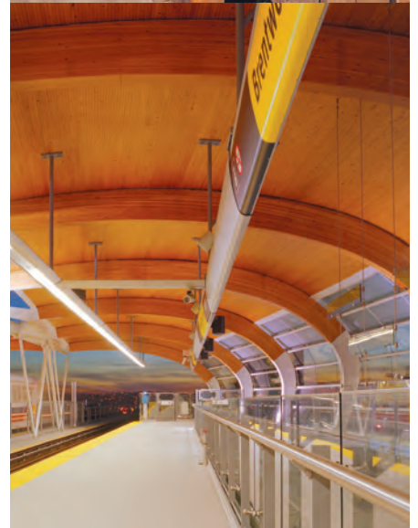
Locally sourced and milled timber used in Millennium Line station canopies.
