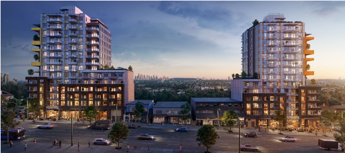
Figure 1. PCI East Village Development (Yarrow on the right)
